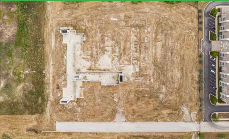
Foundation, flat work, and elevator shafts in place
